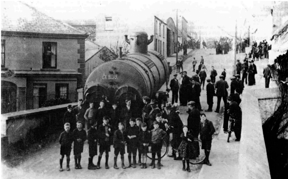
FIGURE 5: THE ARRIVAL OF THE STEAM BOILER 1937 [14]
