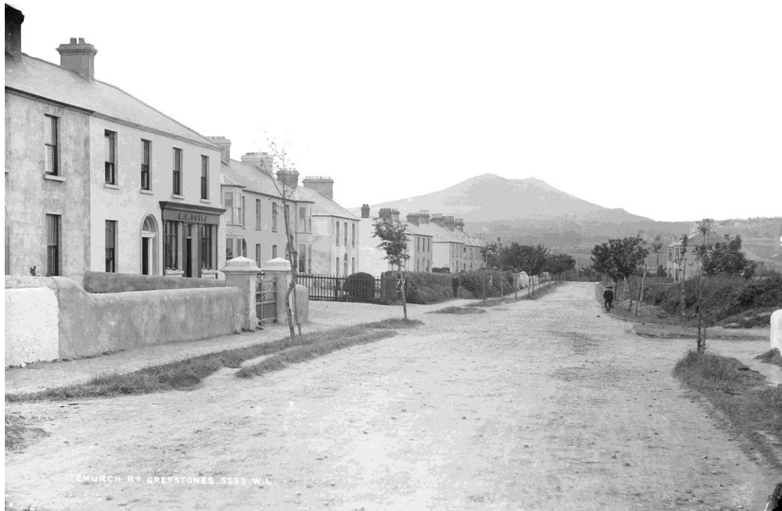
3332.W.L. Shows Enright Doyle's shop on the Church Road, just opposite the junction with Bridge Road.. The road surfaces are unpaved, the standard trees planted in the verges are very immature. I believe this is part of the 1880-ish sequence.
