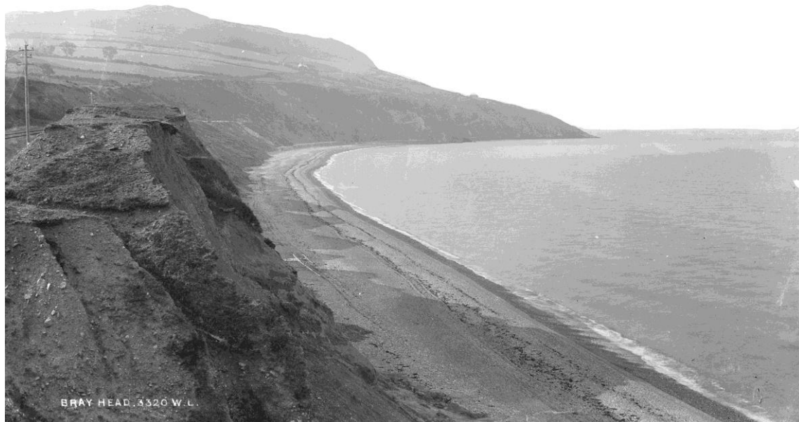
3320.W.L. Bray Head, a photograph of the severely eroded cliffs between Morris's Road and the original 'Gap Bridge' are two images I've dealt with at some length in the Cúl of the Rock paper. Both are part of the sequence.
