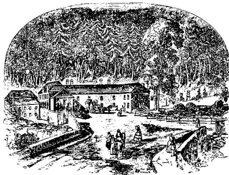
WOODEN BRIDGE HOTEL, COUNTY WICKLOW.
